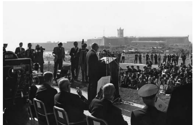
The opening ceremony for IBERLANT, the first permanent NATO command in Portugal. The ceremony was moved outside the walls as a result of the damage from a bomb planted by communist terrorists the night before.
