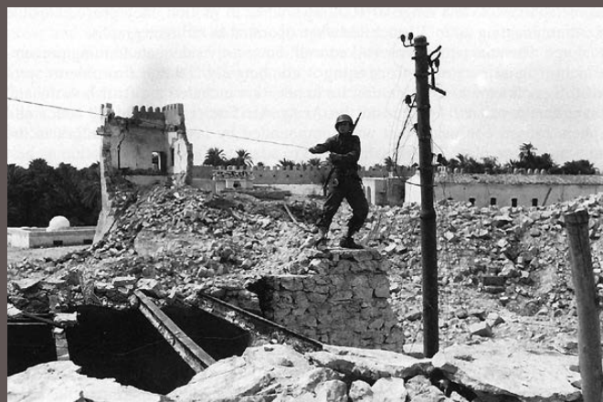
In a denied environment, communications may depend on tried-and-true systems like the field telephone and the soldiers needed to lay its cables.
