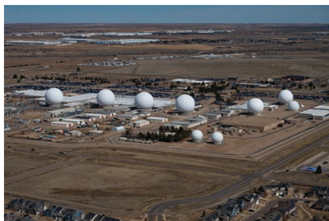
The ground segment is just as important as what's in orbit. At Buckley Space Force Base in Colorado, satellites are controlled and updated, and their information is processed.
