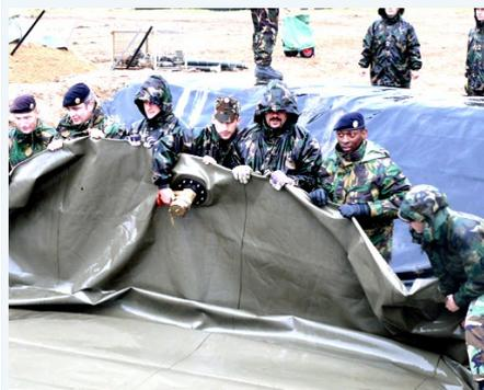
Setting up of a fuel bladder to ensure the continuous fuel supply of an Operation.
